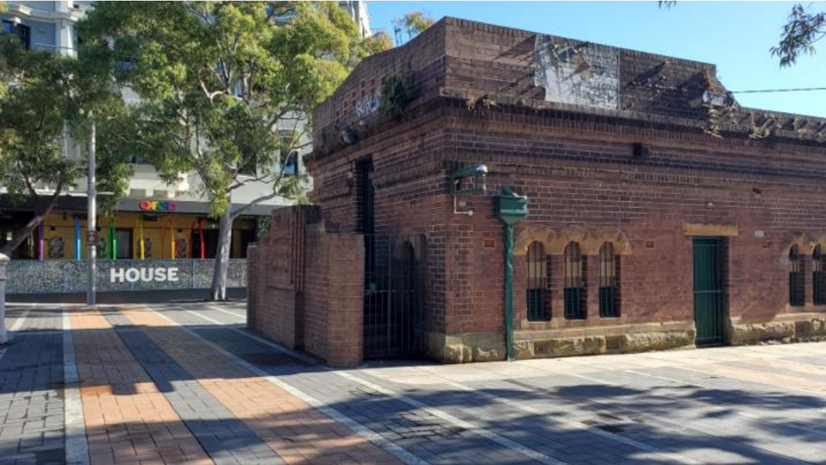
Figure 10: Detail view of substation facing west
