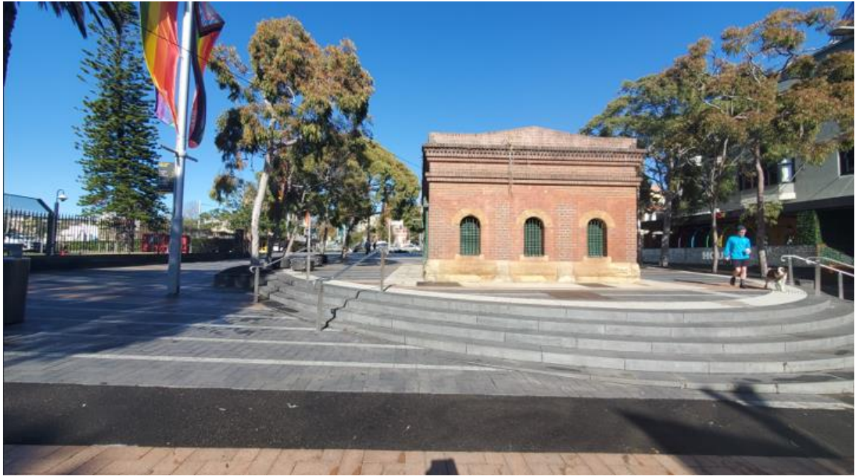
Figure 7: Taylor Square substation facing south
