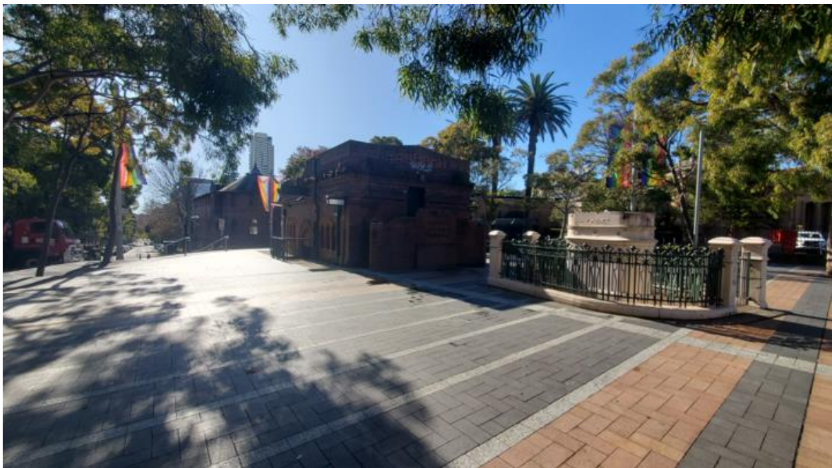
Figure 2: Taylor Square heritage listed substation facing northeast
