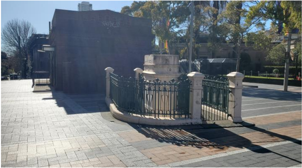
Figure 17: Detail view of entrance to heritage listed underground lavatory, facing northeast
