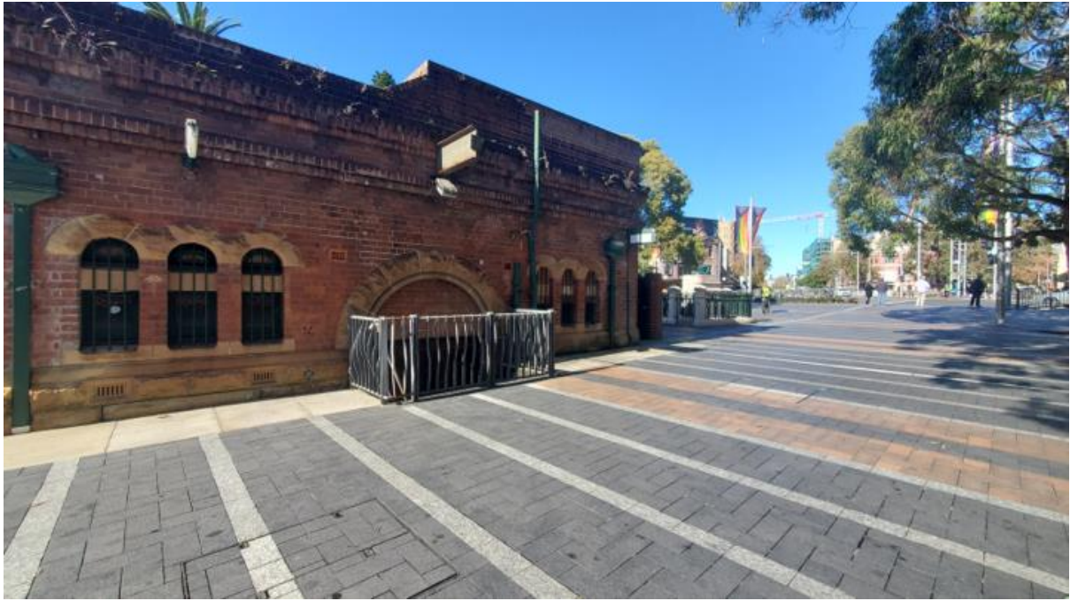
Figure 5: Detail view of substation facing southeast
