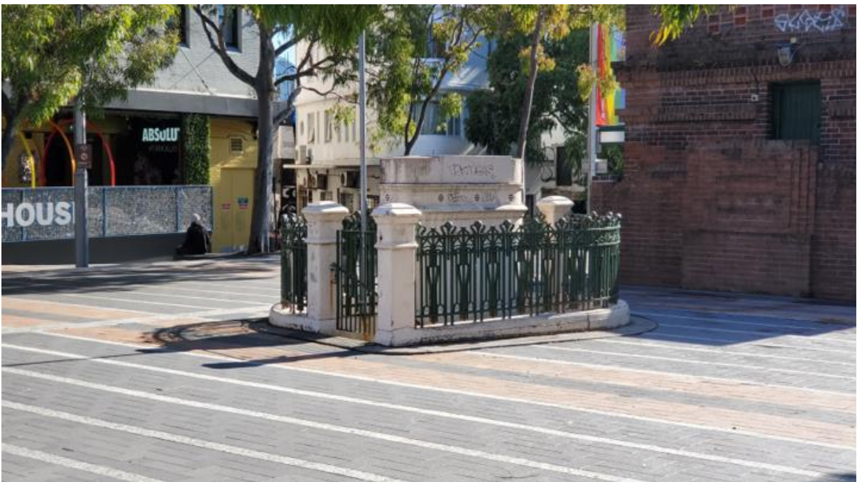
Figure 16: Detail view of entrance to heritage listed underground lavatory, facing northwest
