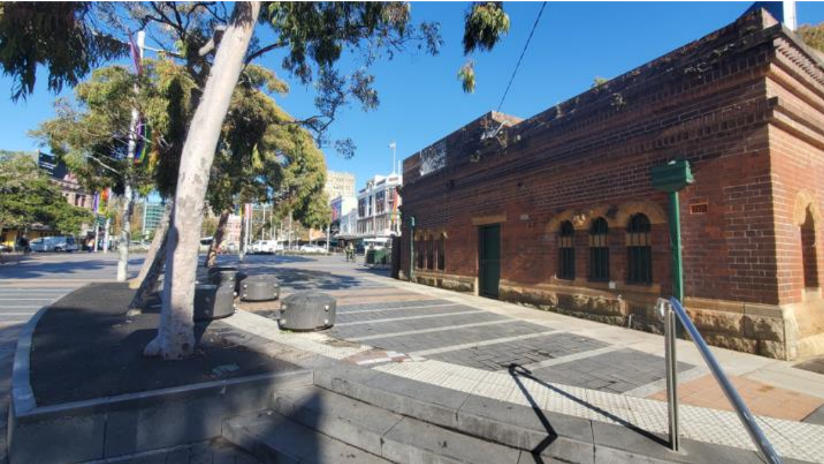
Figure 9: Detail view of substation facing southwest
